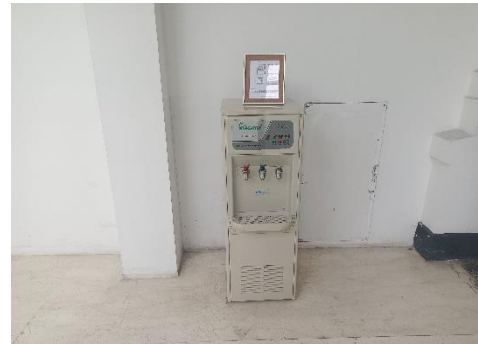
Water Fountain di Gedung H
