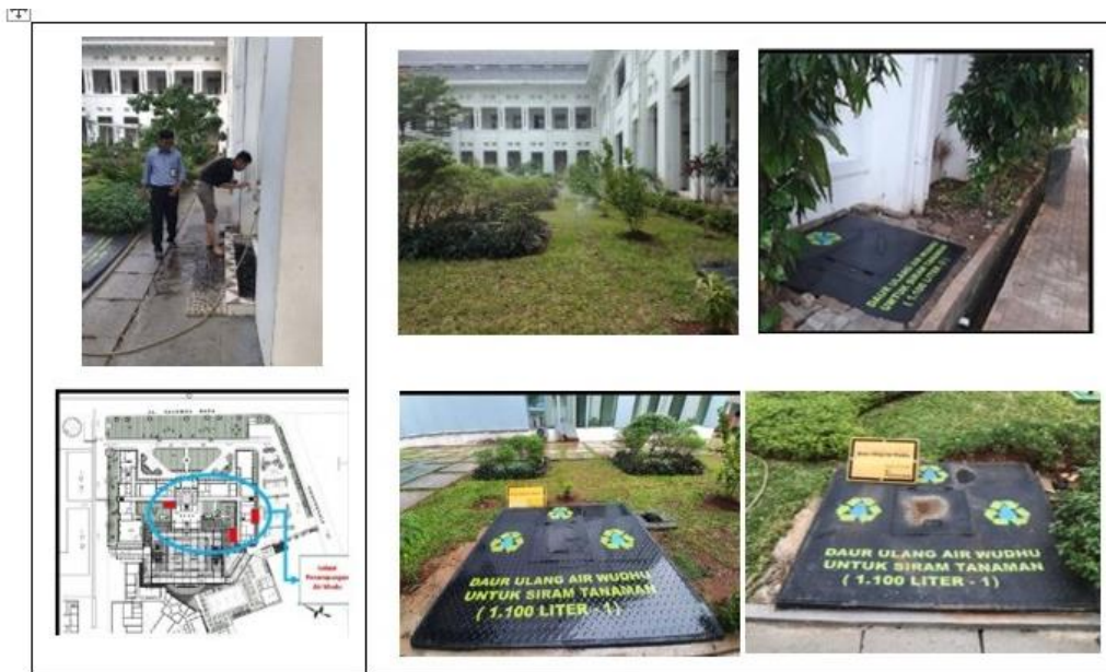
Scheme for Used Ablution Water (Air Wudhu) Recycling
