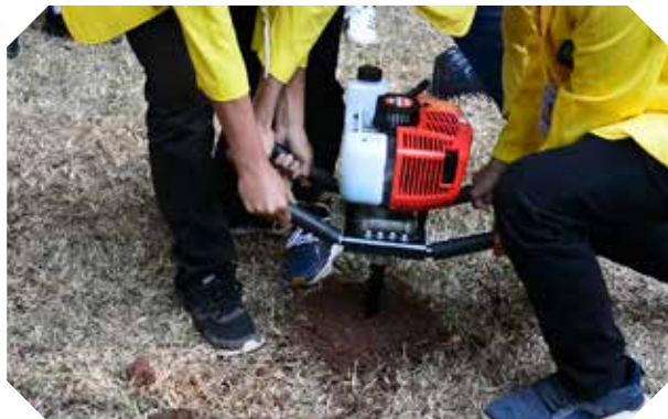
Pembuatan lubang biopori di area kampus. Making biopore infiltration holes on campus.
