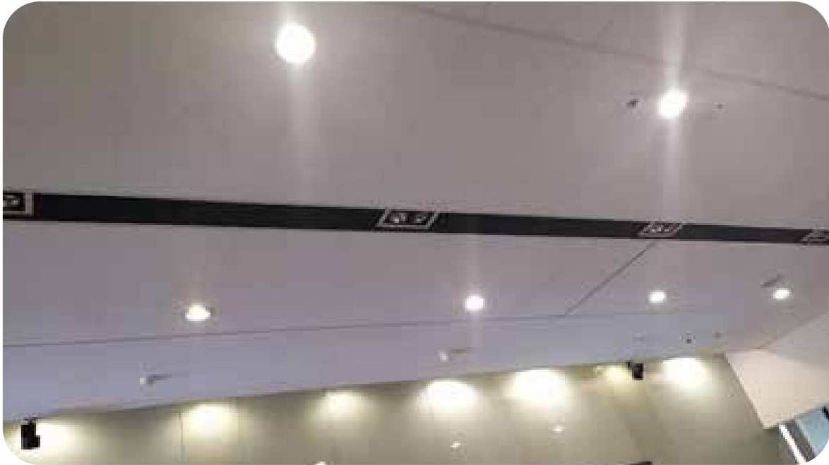
Sistem Pencahayaan LED Sensor Gerak di Gedung Pusat Administrasi UI Motion Sensor LED Lights System at the University Administration Center Building
