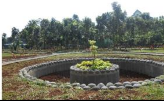
Kolam resapan air hujan di Taman ENG Park.
