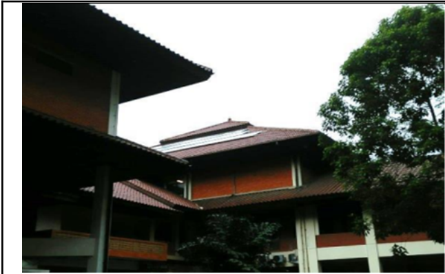
Solar Power Plant Faculty of Social and Political Sciences
