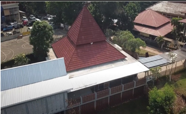
Solar Power Plant of Prayer Room Faculty of Engineering
