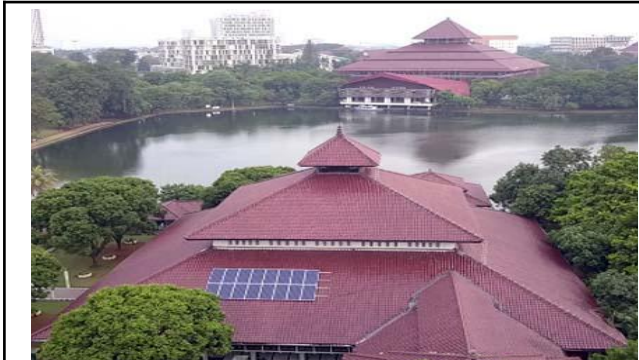
Solar Power Plant UI Mosque
