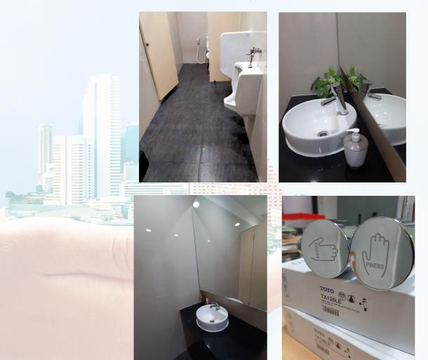
Picture: Utilization of Water-Saving Devices
