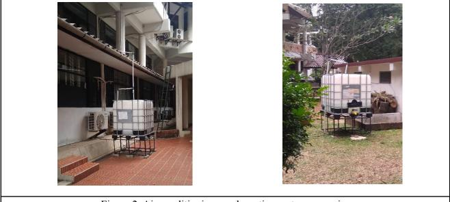
Figure 2. Air conditioning condensation water reservoirs
