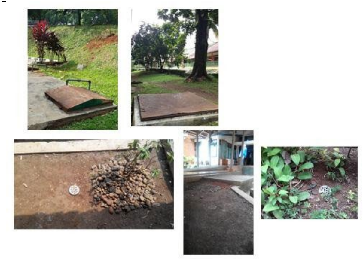
Biopori and Rain Ground Tank System
