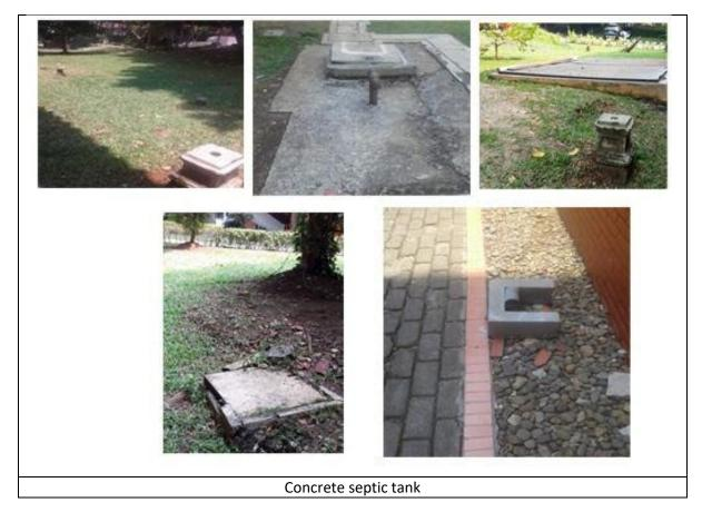
At the Faculty of Psychology, the liquid waste is disposed through a concrete septic tank. This concrete is used to prevent any possible leakage to the ground around it and polluting the water system inside the ground.
